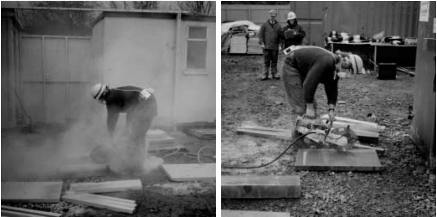
(a) (b) Figure 2 Slab cutting with mains supply water system: (a) without control; (b) with control
