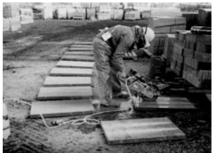
(a) (b) Figure 1 Slab cutting with pressurised portable tank system: (a) without control; (b) with control
