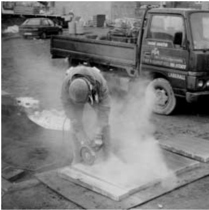
(a) Figure 3 Slab cutting using LEV: (a) without control; (b) with control
